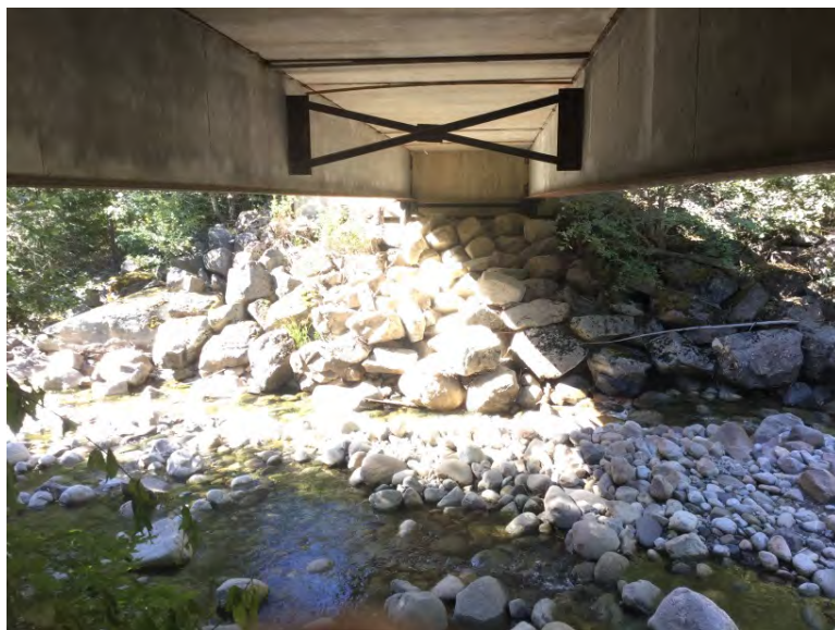
Right Bank Abutment when facing downstream
