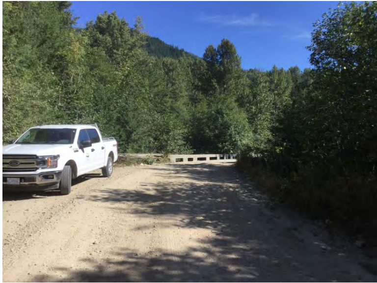
Approach from Right Bank when facing downstream
