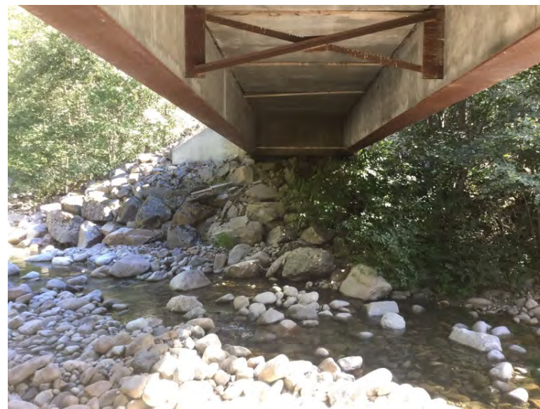
Left Bank Abutment when facing downstream
